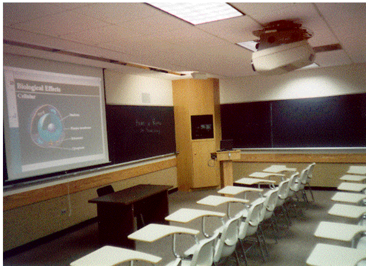
Example of a smart classroom - This angle shows the ceiling mounted video/data projector, the recessed technology control panel and the lectern at the front of the room.
